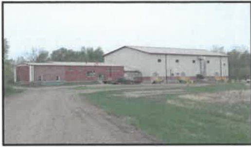
Figure 1. Water Treatment Plant #1
