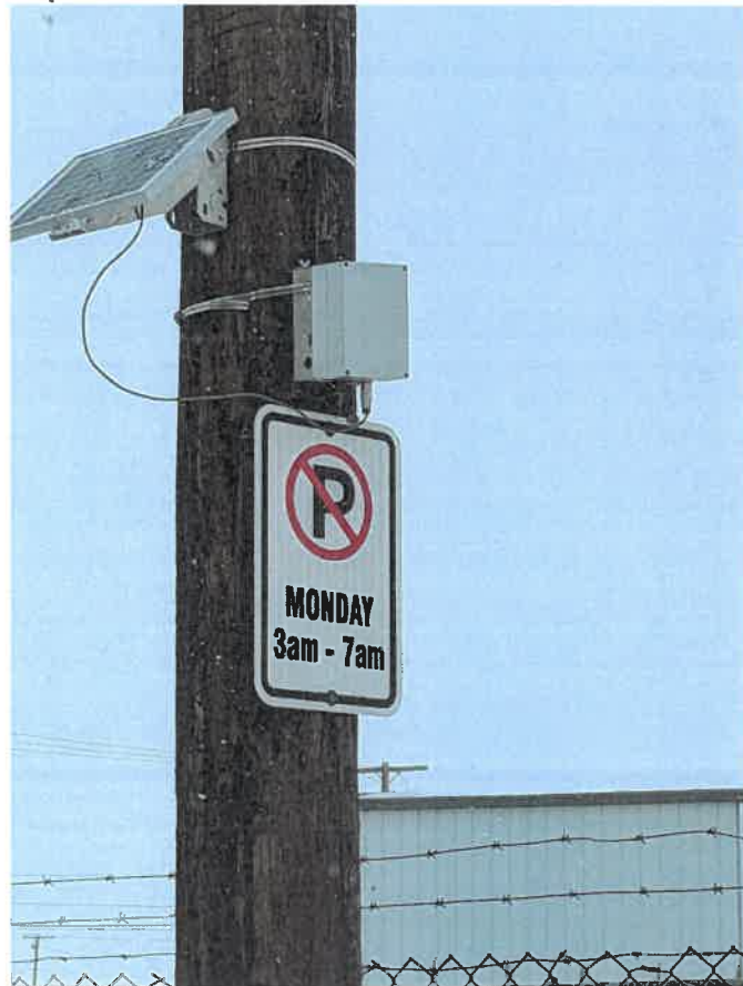
Traffic Counter Mounted on a Power Pole
