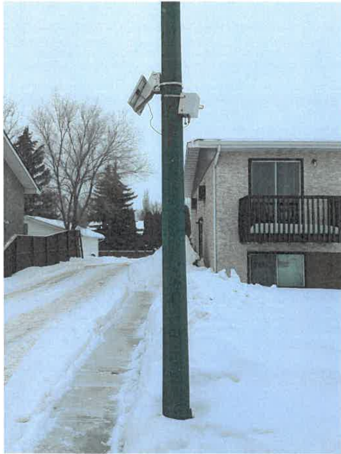
Traffic Counter Mounted on a Streetlight
