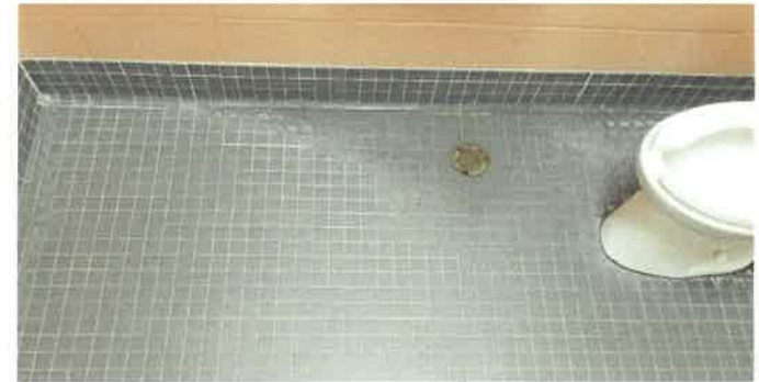
Grout is discolouring due to cleaning products, chlorine and age.
