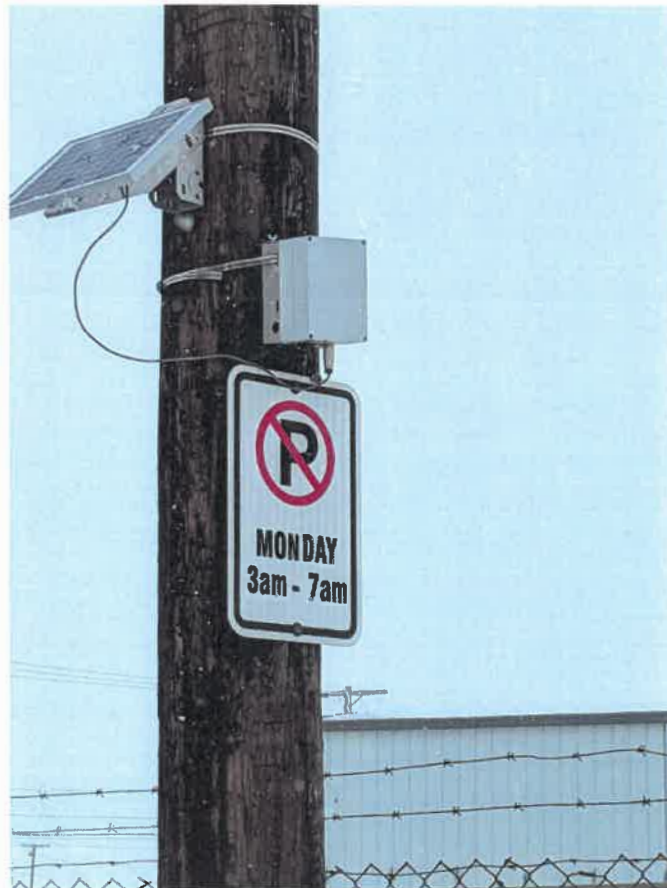
Traffic Counter Mounted on a Power Pole
