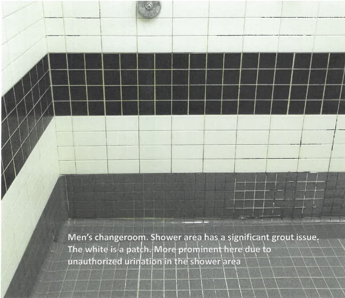
Grout is discolouring due to cleaning products, chlorine and age.
