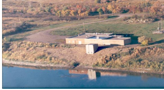
Figure 2. F.E. Holliday Water Treatment Plant
