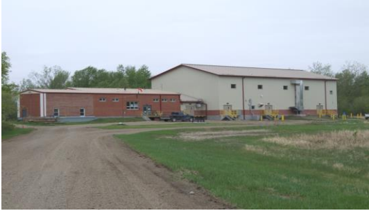
Figure 1. Water Treatment Plant #1
