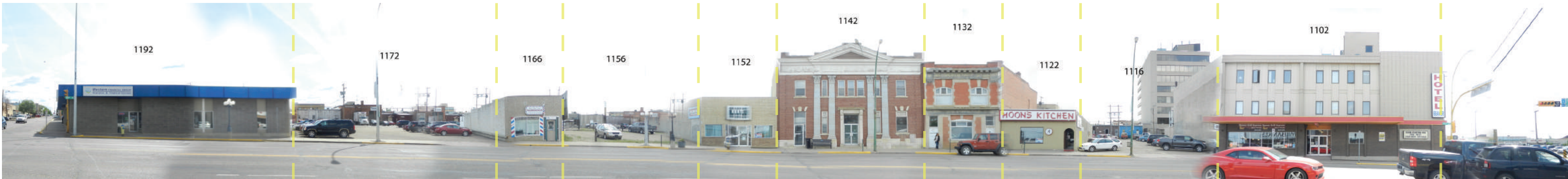
100th Street 1100 Block EAST 18/06/2015
