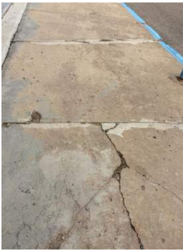
North end sidewalk
