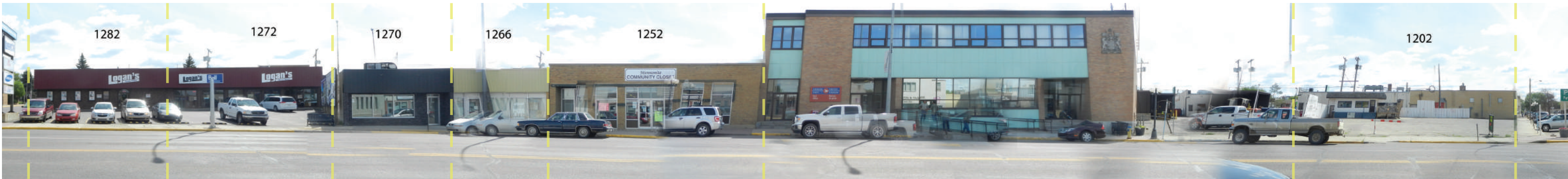
100th Street 1200 Block EAST 18/06/2015
